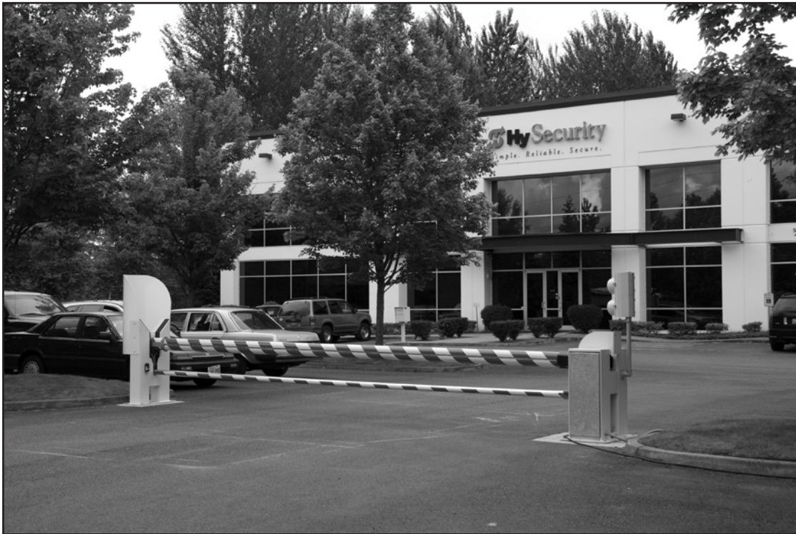
HySecurity Gate, Inc. Headquarters in Kent, WA
