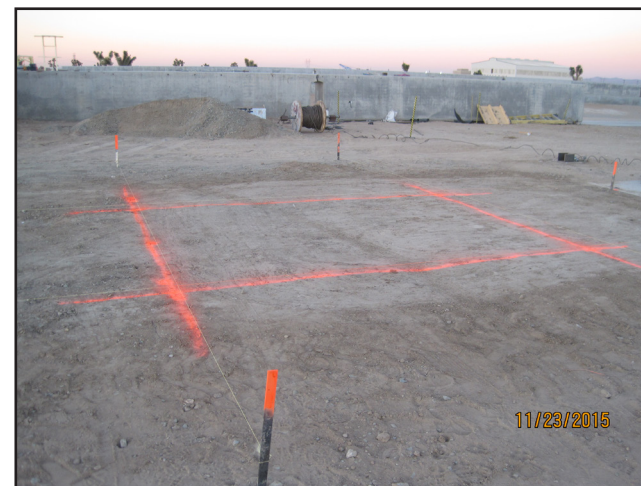
Designate site layout for resurfacing
