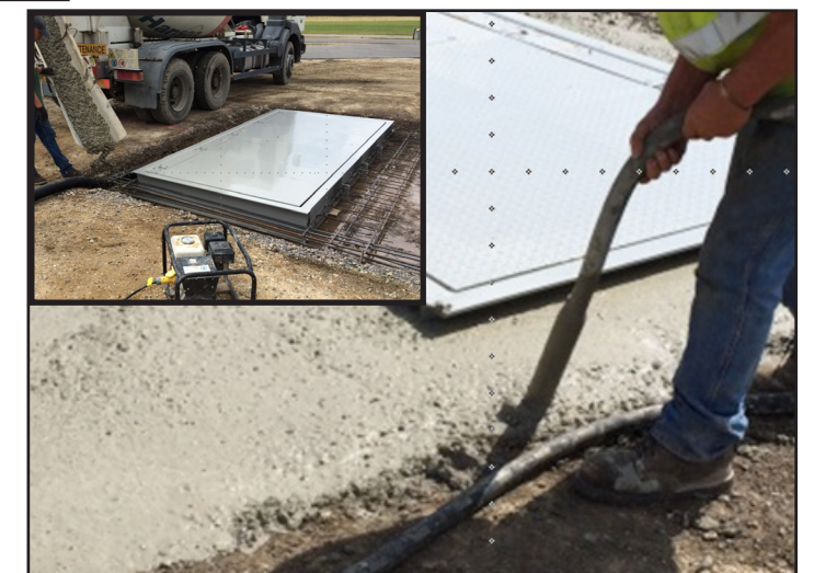
Remove air pockets. Smooth and finish.
