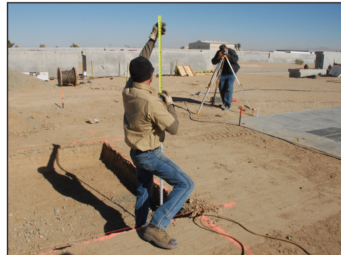
Survey site location. Verify depth to grade
