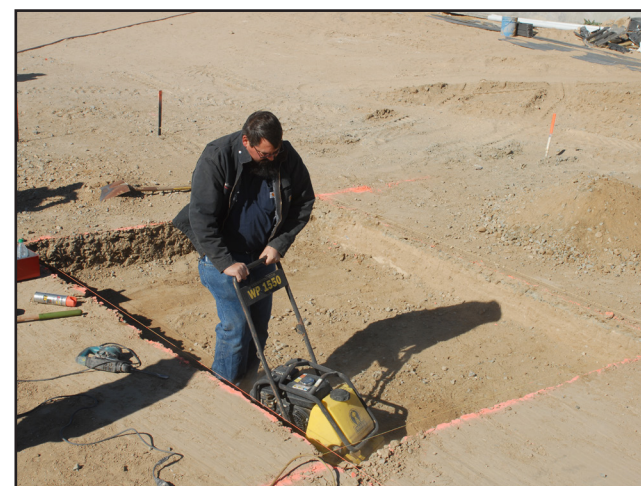
Compact soil and prep drainage channels
