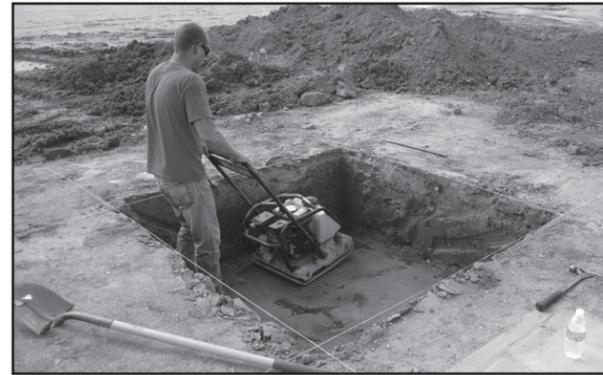
Soil Density compacted to 95% per ASTM-698
