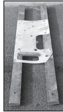
Example Concrete Template Chassis base & conduit
