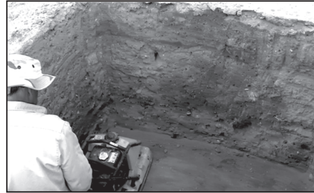
Soil Density compacted to 95% per ASTM-698
